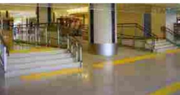
Figure 7-8: Placement of warning blocks for steps
