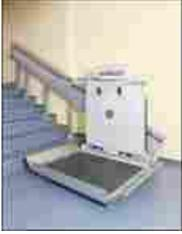
Figure 7-18: Platform chair lift and platform lift
