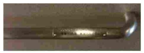
Figure 5-25: Handrail with Braille Information Panel
