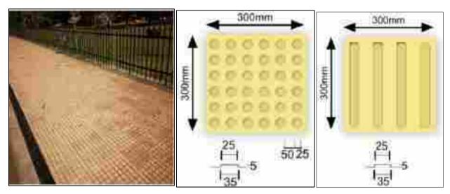
Figure 5-1: Chequered tile on footpath
